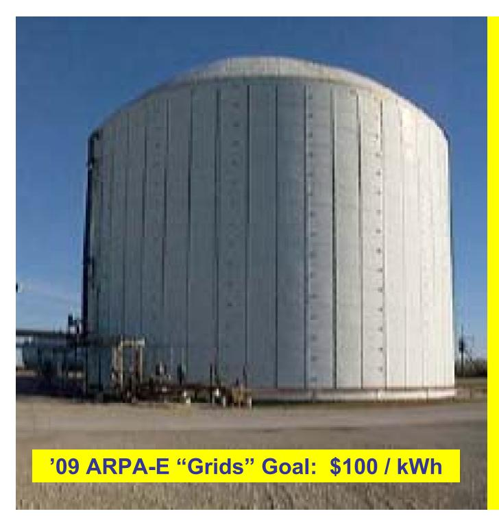
"Atmospheric" Liquid Ammonia Storage Tank (corn belt) 30,000 Tons 190 GWh
