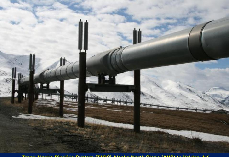
Trans Alaska Pipeline System (TAPS) Alaska North Slope (ANS) to Valdez, AK tanker loading terminal. Design capacity: 2 million barrels / day crude oil
