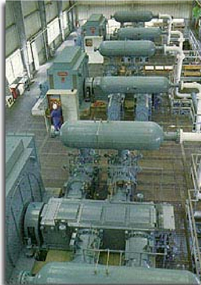
Three 8500 horsepower HHE-VL units compress natural gas to 2700 psi into underground storage caverns.
